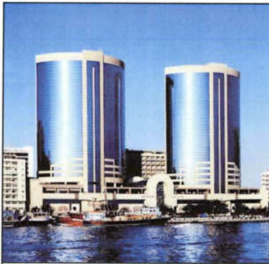
The Twin Towers, Dubai fitted with PX200 using Schüco Profile
